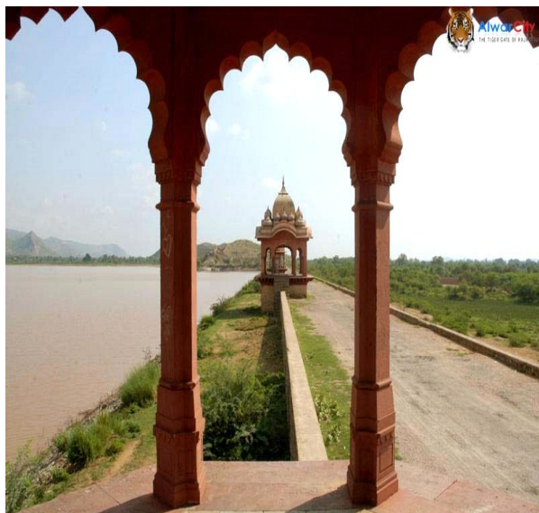
Fig 3: Pavilion towers erected on dam of the lake.
