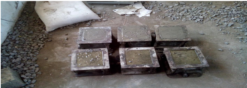
Figure.1 – Casting of Specimens
