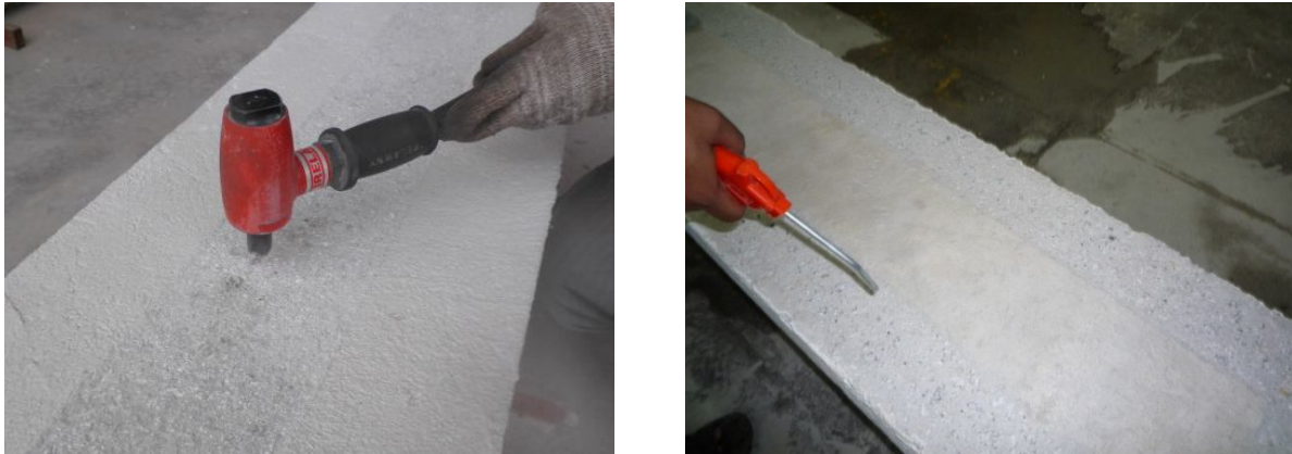
Figure 1: Preparation of surface
