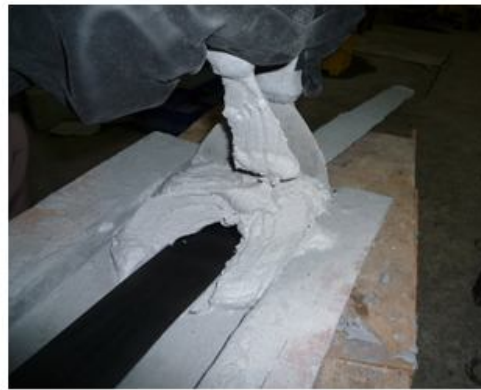
(b) Placing of adhesive on CFRP laminate
