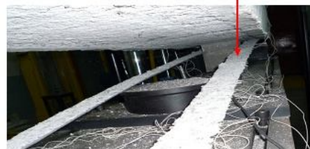
Figure 6: Failure mode of beam B6
