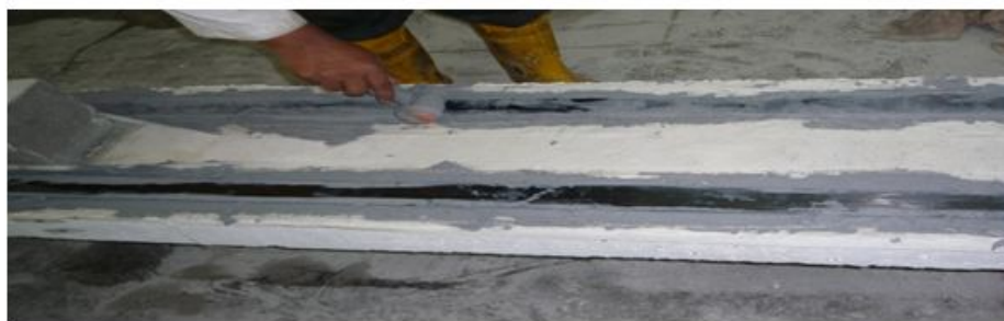
(c) Pressing CFRP with the help of Rubber Roller
