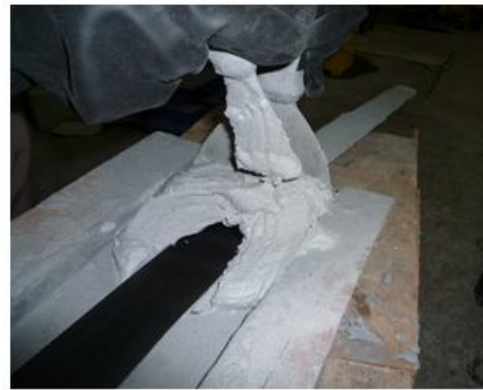
(b) Placing of adhesive on CFRP laminate
