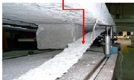
Figure 7: Failure mode of beam B7
