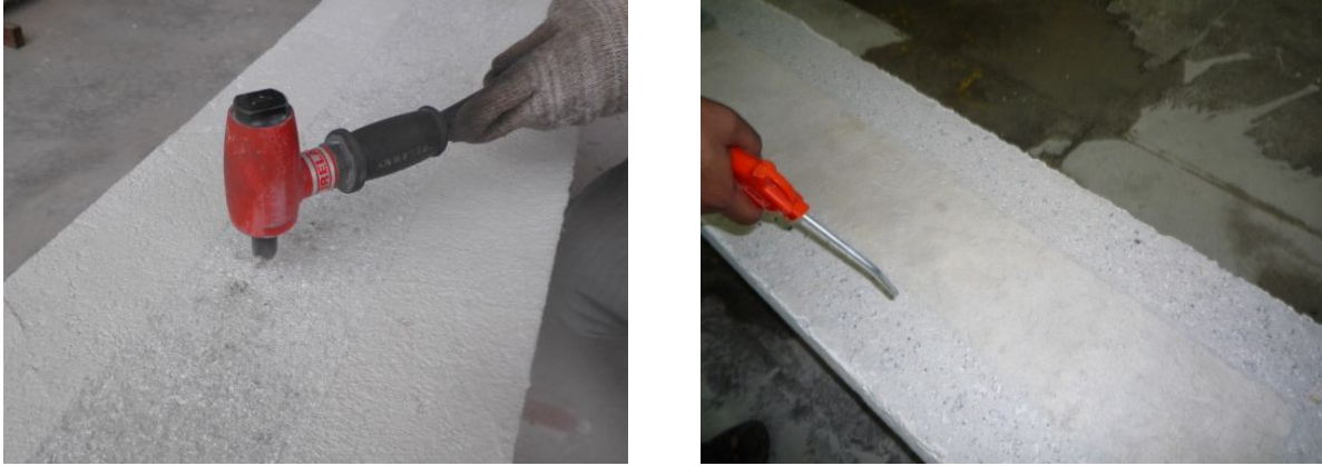
Figure 1: Preparation of surface
